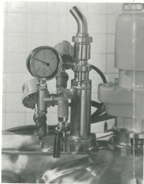
Pneumatically operated vacuum and ventilation valve, relief valve and manometer.
